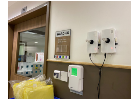
External Alarm Unit placed outside the isolation ward is triggered to alert nurses
